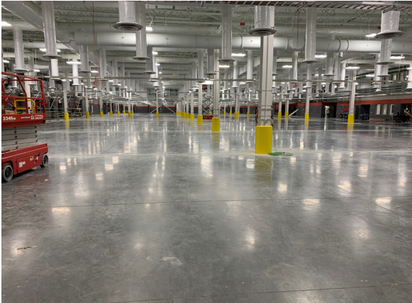
WCF Expansion Project: West production area
