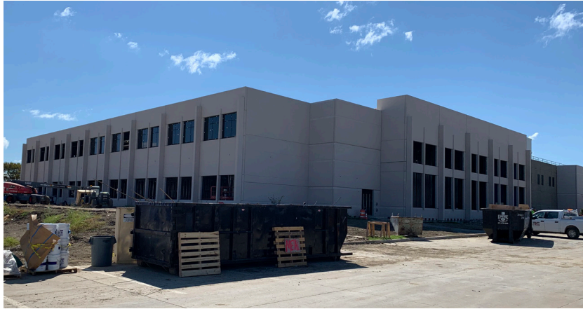
WCF Expansion Project: Exterior of administrative addition
