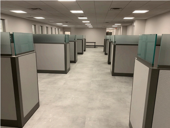
WCF Expansion Project: Interior of administrative addition
