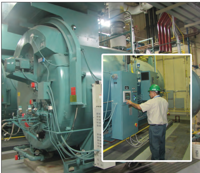
The WCF's Boiler Room contains three new, energy-efficient boilers. Inset: A contract maintenance worker monitors the equipment.
